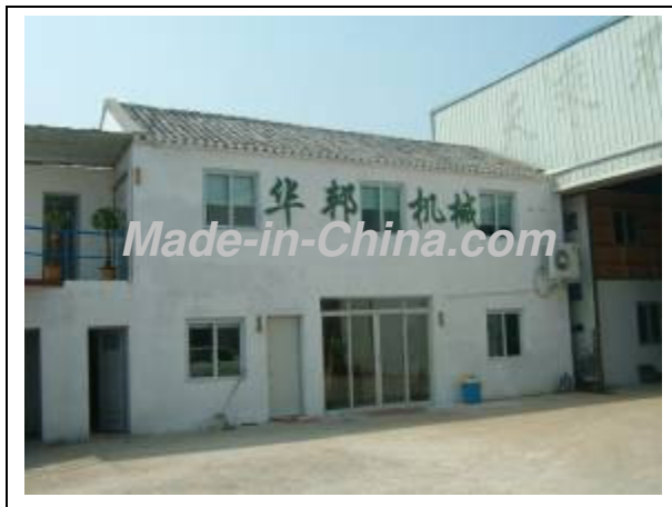
Description: Office building
